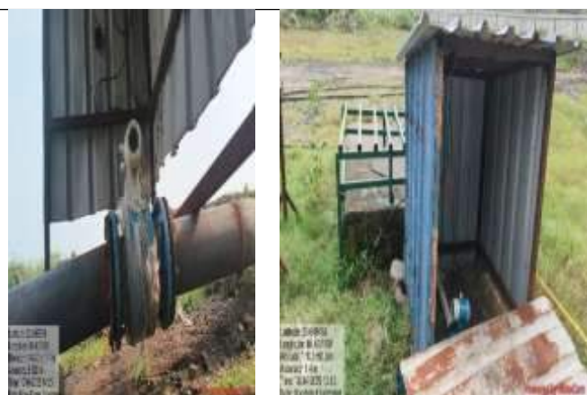
Flowmeters installed at the mines area
