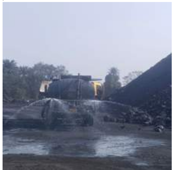
Dust Suppression by Water Sprinkling
