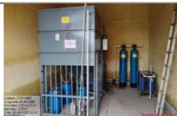
Effluent Treatment plant installed at Project site
