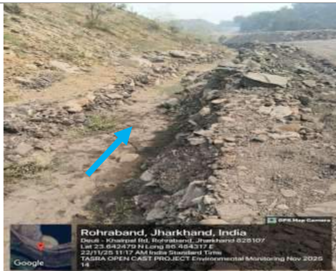
Catch drain near the dump area
