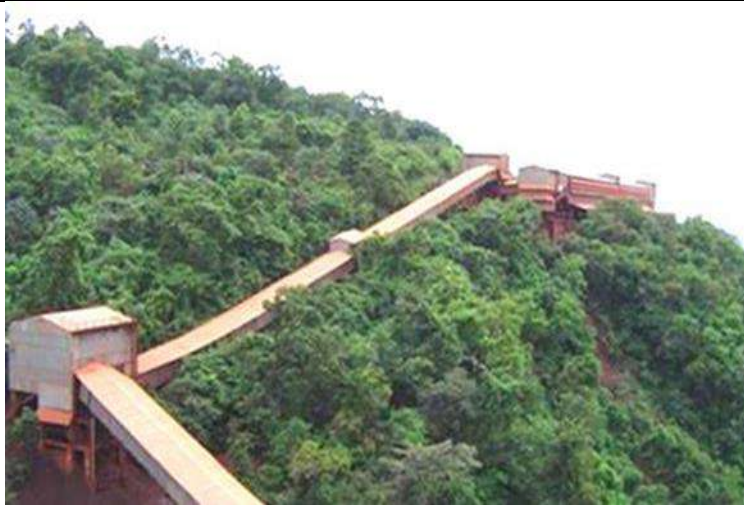
Covered conveyors from Mines till dispatch point
