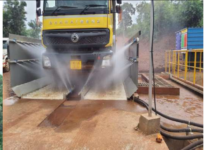
Wheel Washing System Installed at Exit Gate of Fines Selling Area
