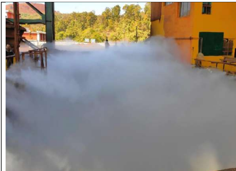
DFDS Installed at Feed Hopper of 1600 TPH Plant
