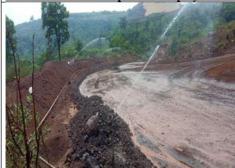
Fixed Sprinkler Installed at Permanent Haul Road of FandG Area
