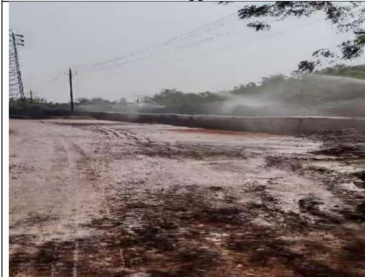
Fixed Sprinkler Installed at Roads Around Loading Plant
