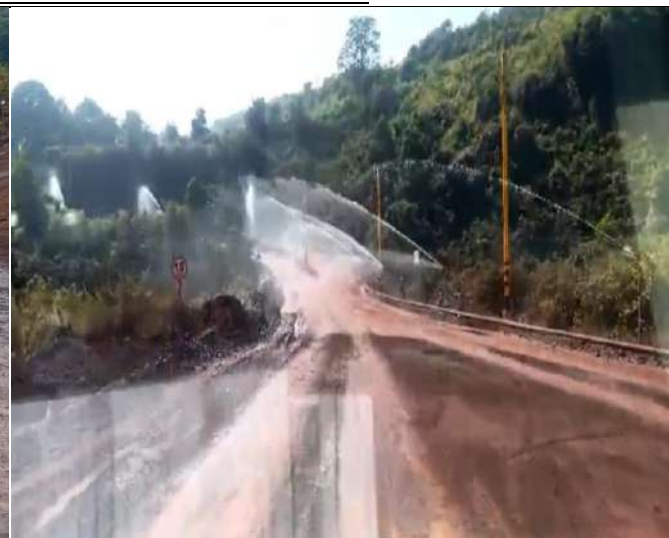
Fixed Sprinkler Installed at Permanent Haul Road of D and Panposh Area
