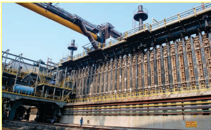
The newly built COB #11 of ISP, with 74 ovens, each 7 meter tall, having an annual production capacity of 0.882 MTPA
